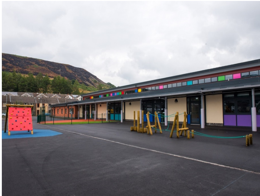
External view of Cwmaman Primary School opened by The Council in 2018.
